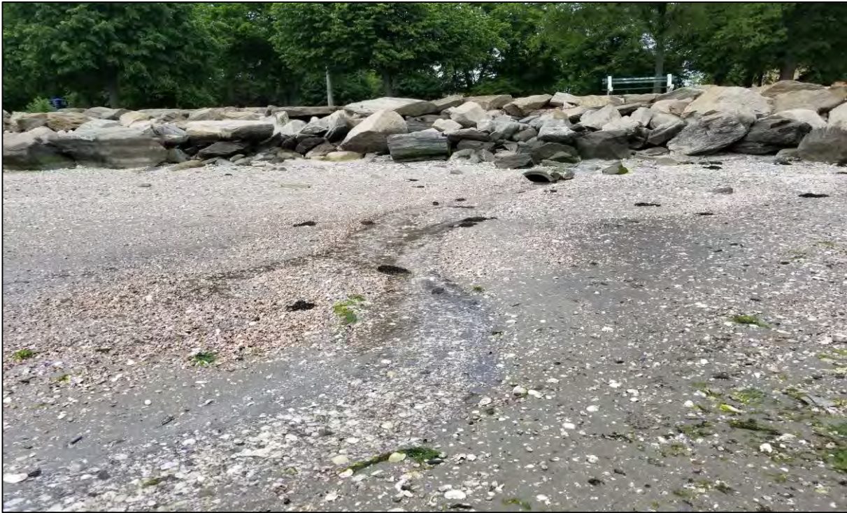
PHOTO 1: Existing Outfall A, partially buried, looking west towards Seaside Park.
