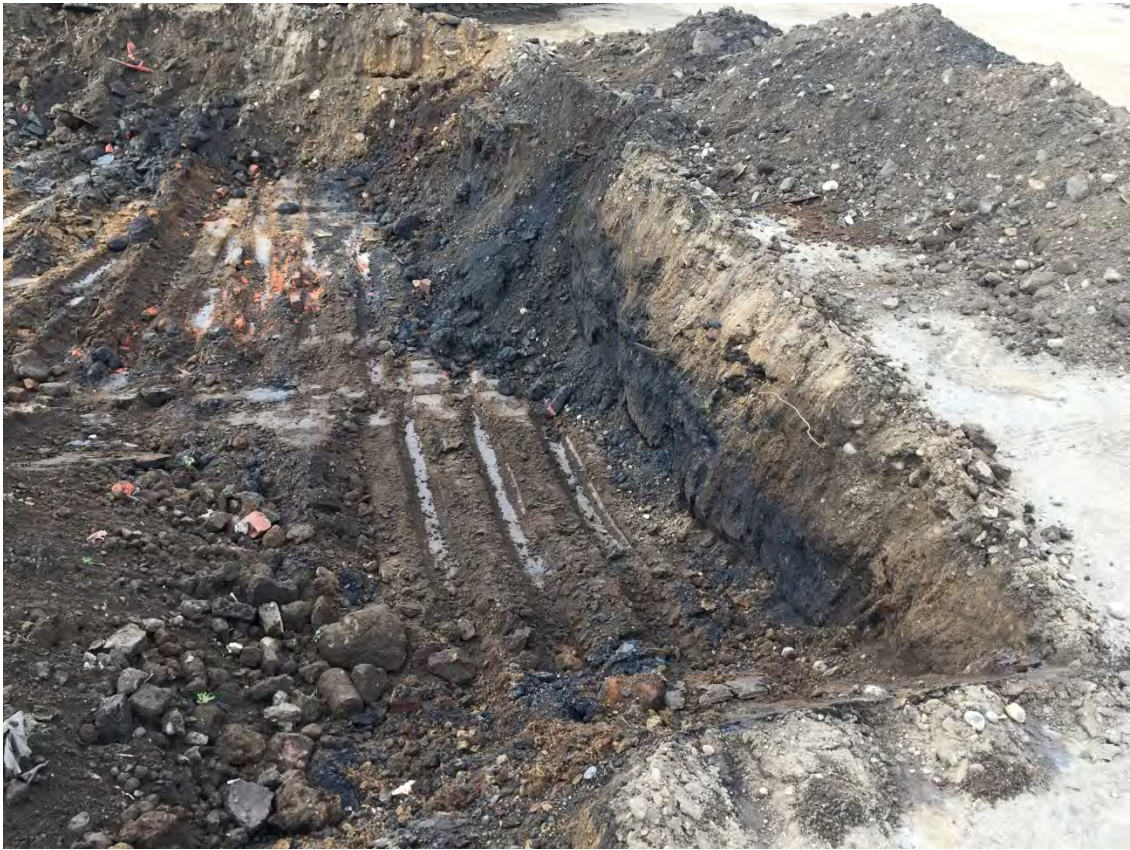
Photo 3: Removal of material from coal storage area
