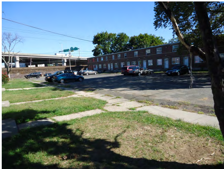
Photo 10: View of parking lot at the east end of the site.
