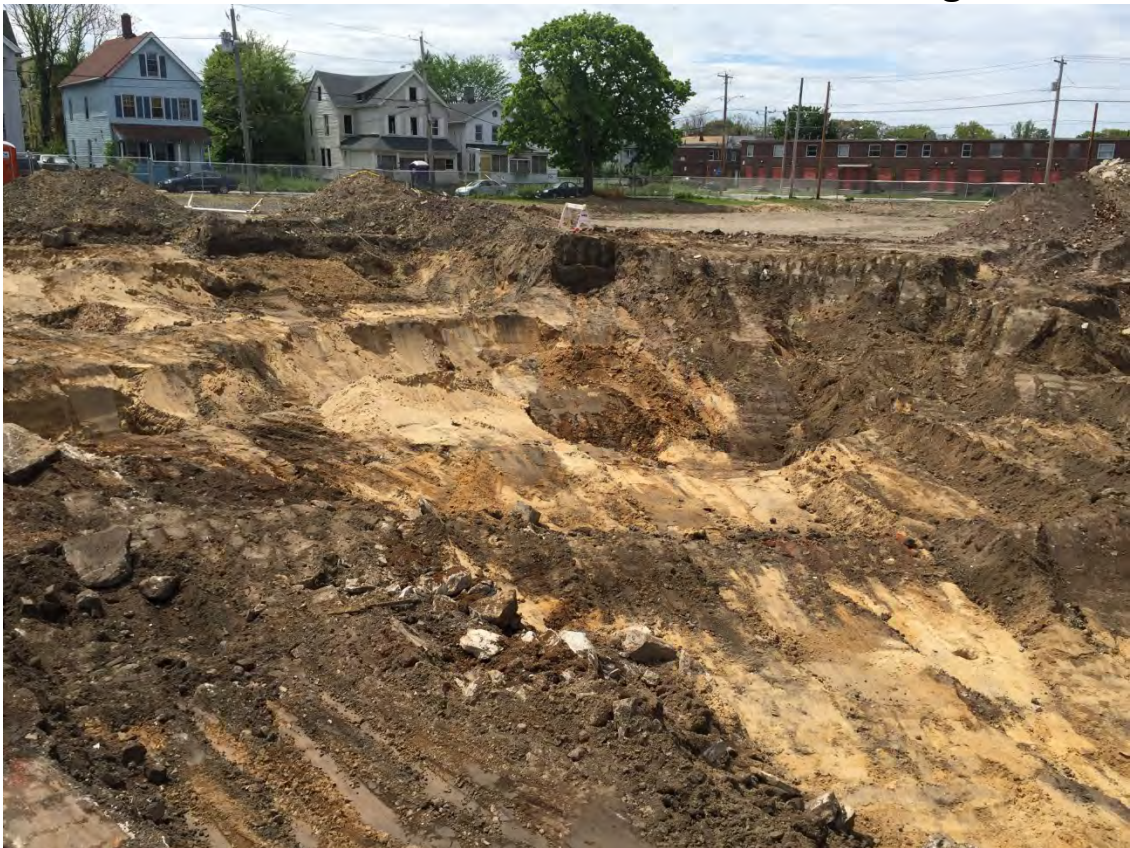
Photo 4: Clean sand remaining after removal of impacted material
