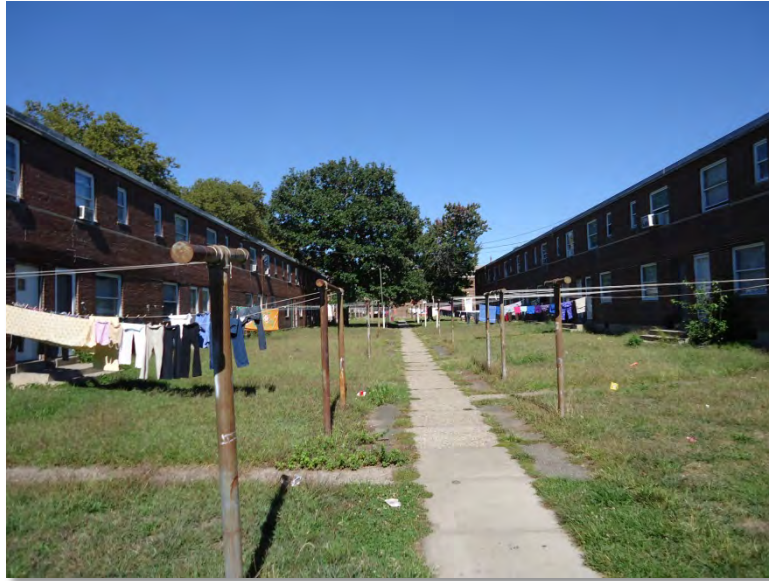
Photo 9: View of courtyard between buildings.
