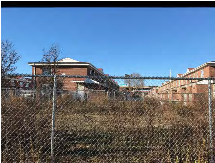
View of Buildings 20 and 21 located at the southern portion of the RBD Pilot Area looking to the northwest.
