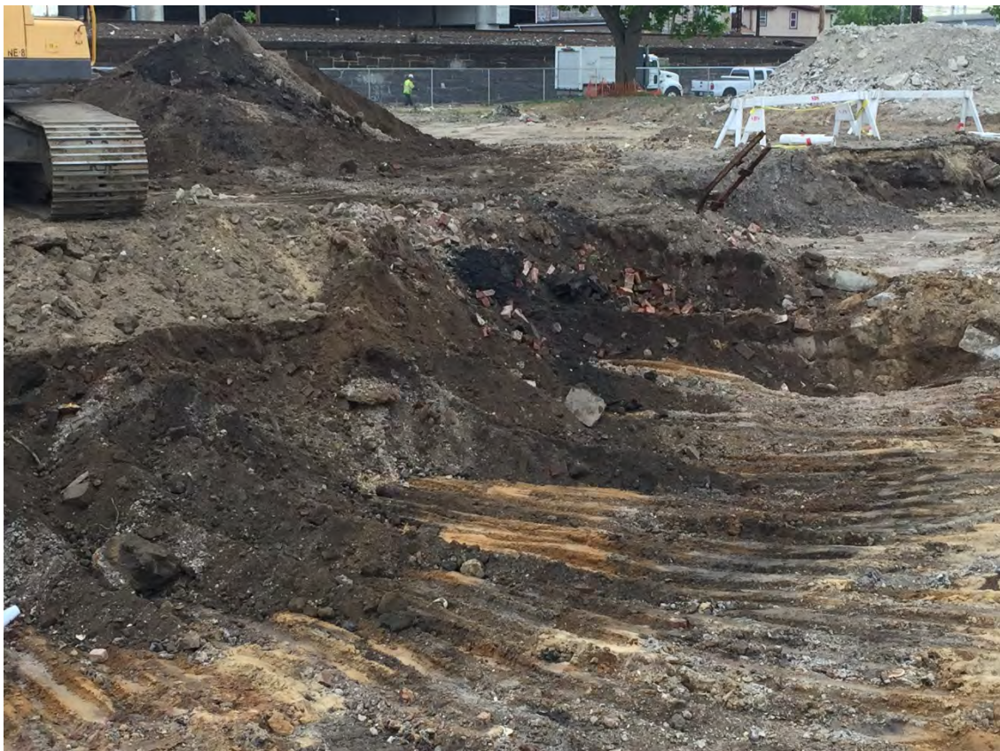
Photo 2: Removal of ash material
