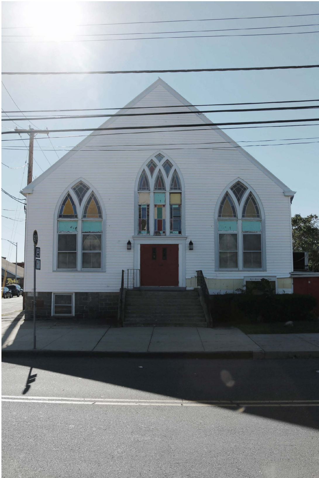
One of multiple Bridgeport South End community centers damaged and unrepaired after Hurricane Sandy
