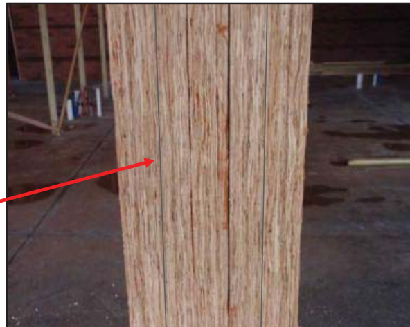
Multi-Ply Nailed Columns ≠ Solid Section
