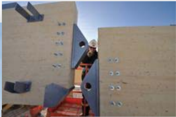
Typical concealed hinge (pinned) connections
