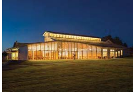
Wood in Educational Buildings Indian Mountain Student Arts & Innovation Center Lakeville, CT Architect: Flansburgh Architects Engineer: Roome & Guarracino Photo: Robert Benson Photography
