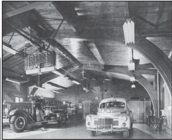
Photos provided by: Structural Wood Corporation
