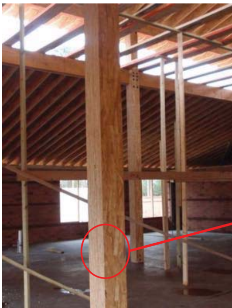
Multi-Ply Columns OK for unprotected Construction
