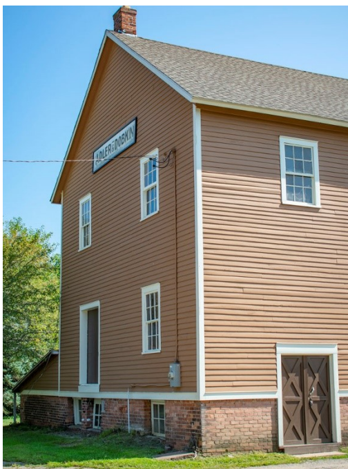
The historic Adler-Dobkin warehouse on Main Street in South Windsor sits on land permanently preserved for agricultural use.
