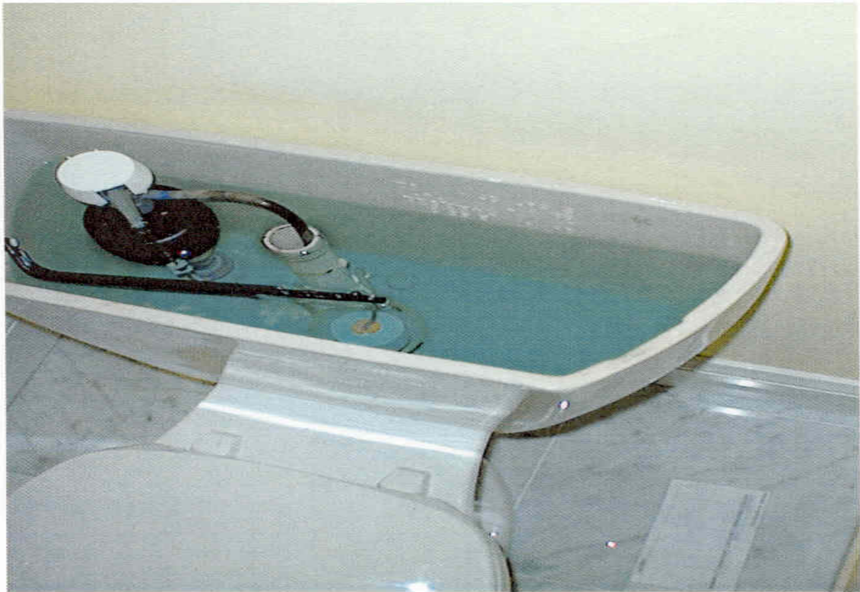
59ppm Copper 3rd floor 47 Cardinal Drive
