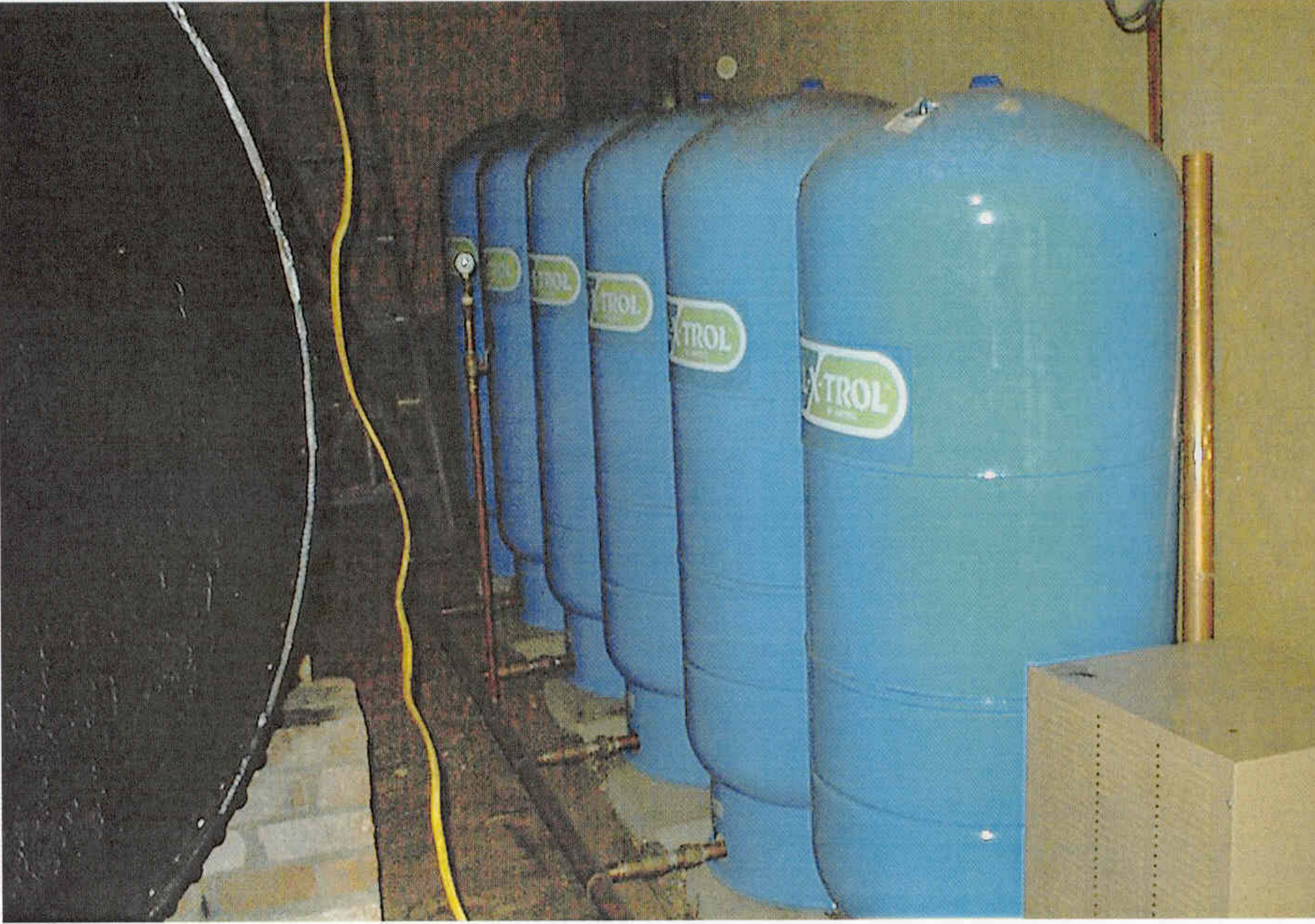
6-Well-X-Trol WX-350 Pressure Tanks, Total Useable Volume @180 gals.
