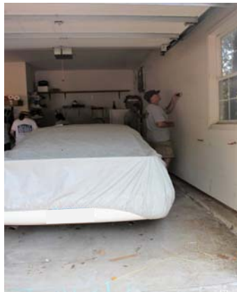
Garage Makeover: Bay 2 – Progress
