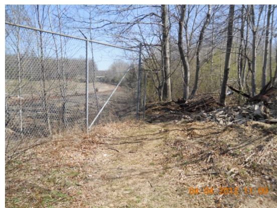
Missing portion of perimeter fence
