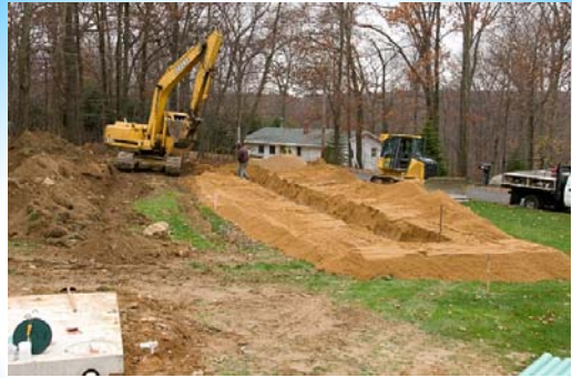
The trench is dug within the compacted fill area
