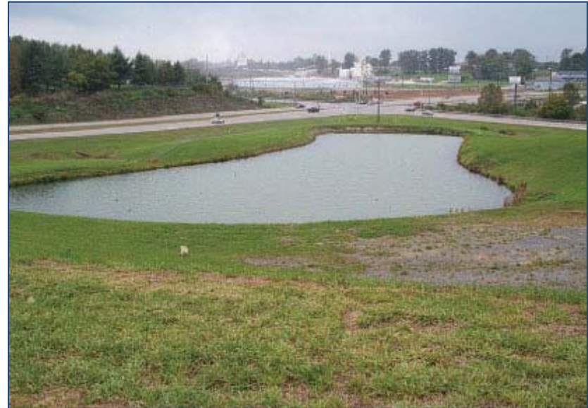
Post-Construction Wet Pond
