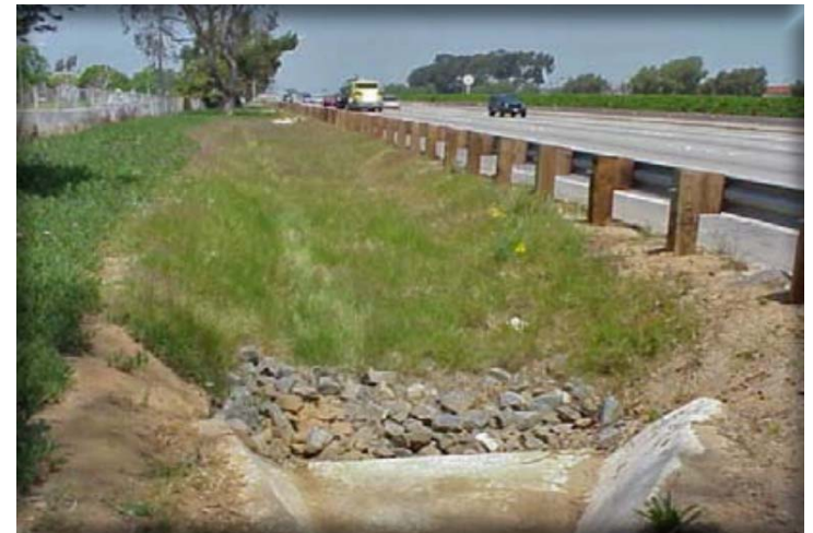
Grassed Channel (Biofilter Swale). Structural BMP Specifications for the Massachusetts Stormwater Handbook. Vol. 2 Chap. 2. Massachusetts Department of Environmental Protection. Retrieved from https://www.mass.gov/files/documents/2016/08/gi/v2c2.pdf
