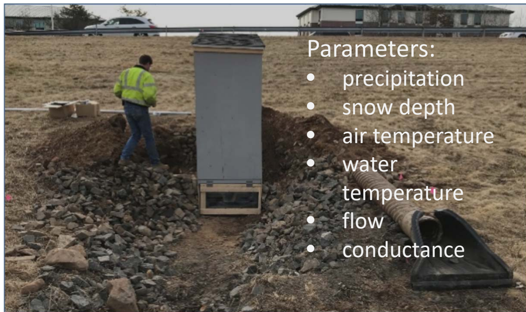
CTDOT Photo of USGS building an outfall monitoring station in Glastonbury
