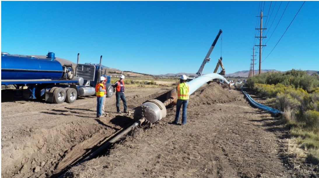
FIGURE 3-12. INTERCONNECTING TWO WATER SYSTEMS
