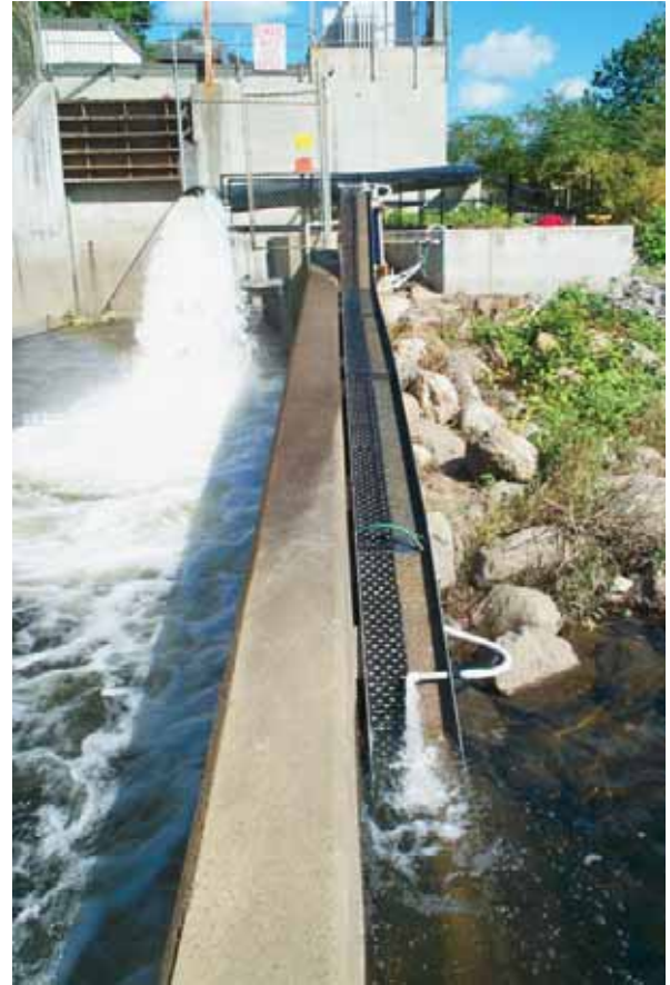
An Irish Elver Ramp in operation in Connecticut. A small amount of water flowing over a rough surface is all the eels need to climb up the pass. Eels slide into a screened trap once they reach the top of the ramp. They are removed each day and released into the river above the dam.
