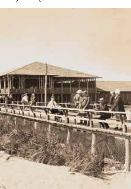
The completed pavilion at Hammonasset Beach State Park drew thousands of visitors who enjoyed the fresh air and walked the 16-foot wide, 1,600-foot long boardwalk. Some even went into the water!
