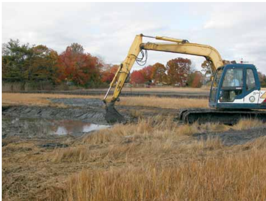
A WHAMM Program excavator digs a shallow pool.
