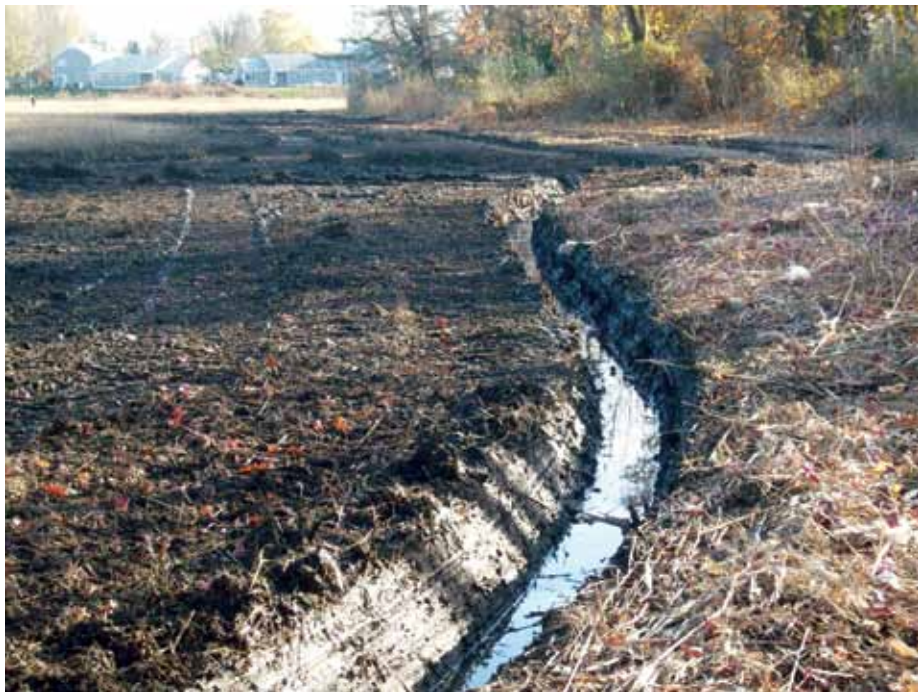
A newly-dug channel shows a thin layer of spoil disposal.
