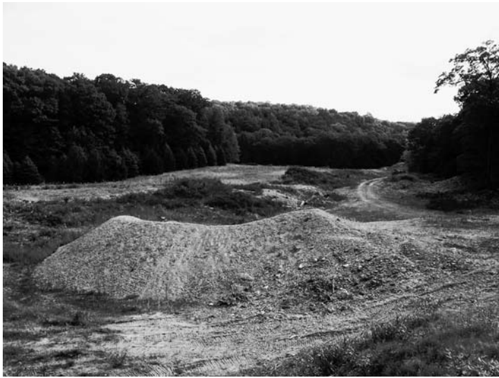
(Left) Several acres of a former 9-acre gravel excavation site at Machimoodus State Park in Haddam will be planted with warm season grasses in spring 2009 using a Truax no-till seeder. (Right) In preparation for the planting, scattered trees and shrubs were removed from the area using a tracked excavator with a heavy-duty, drum-style mowing head (brontosaurus), and the ground was re-contoured using a John Deere 650 bulldozer in September 2008.
