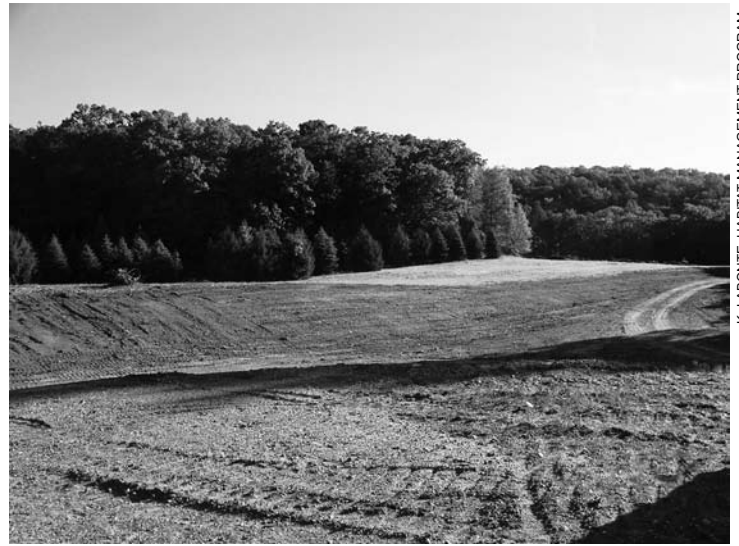
(Left) Several acres of a former 9-acre gravel excavation site at Machimoodus State Park in Haddam will be planted with warm season grasses in spring 2009 using a Truax no-till seeder. (Right) In preparation for the planting, scattered trees and shrubs were removed from the area using a tracked excavator with a heavy-duty, drum-style mowing head (brontosaurus), and the ground was re-contoured using a John Deere 650 bulldozer in September 2008.
