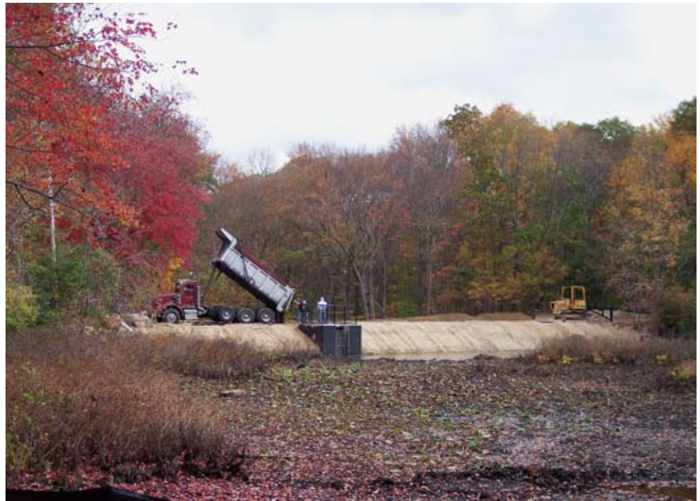
The Northern Dam at Babcock Pond WMA (Colchester) was restored through a cooperative project between the DEP, USDA WHIP, CT Duck Stamp Program, and Connecticut Waterfowl Association. The dam maintains 160 acres of shallow marsh wetlands.
