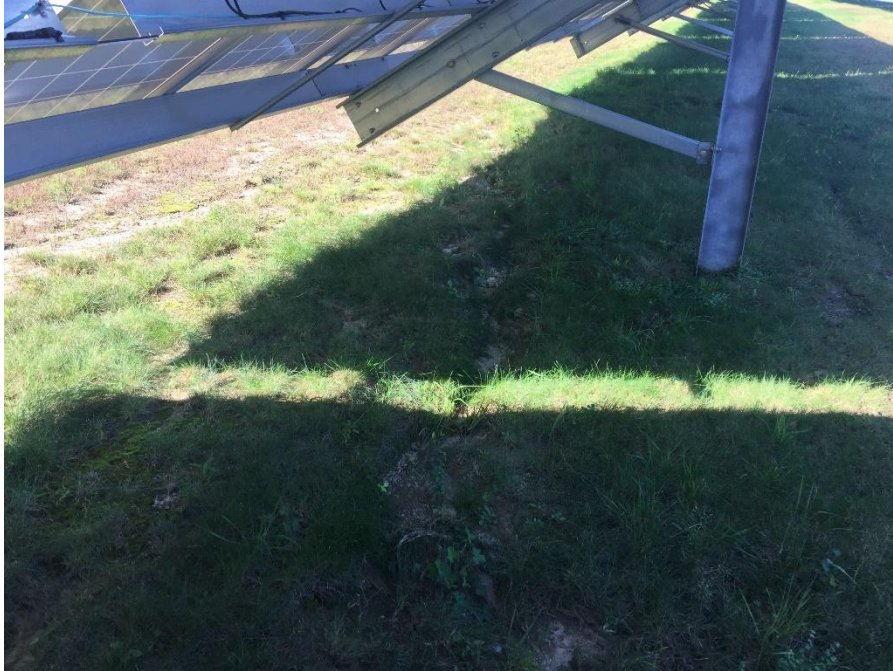
Figure 1 - Concentrated flow from runoff off solar panel
