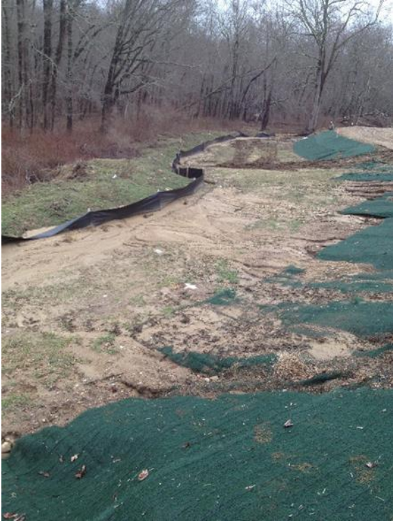
Figure 1 - Erosion Control Blanket (mat)
