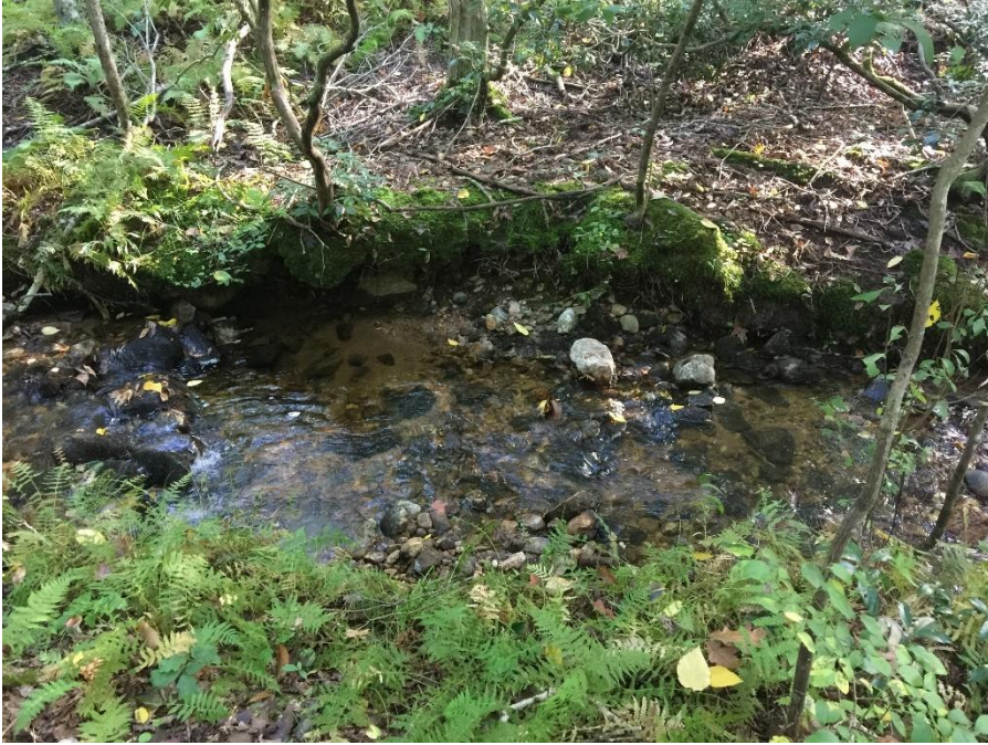
Figure 10 - Undercutting of channel bank of un-named stream on Bialowans Property
