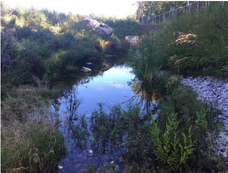
Figure 9 - Wetland Conditions in Bottom of Stormwater Basin
