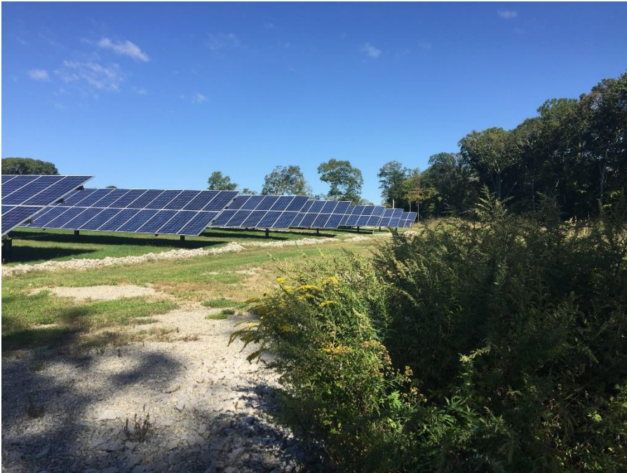
Figure 5 - Stone Berms at downhill end of panel rows
