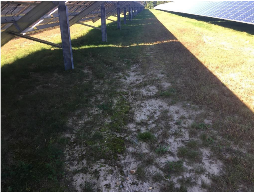
Figure 7 - Erosion & Sedimentation resulting from concentrated flow
