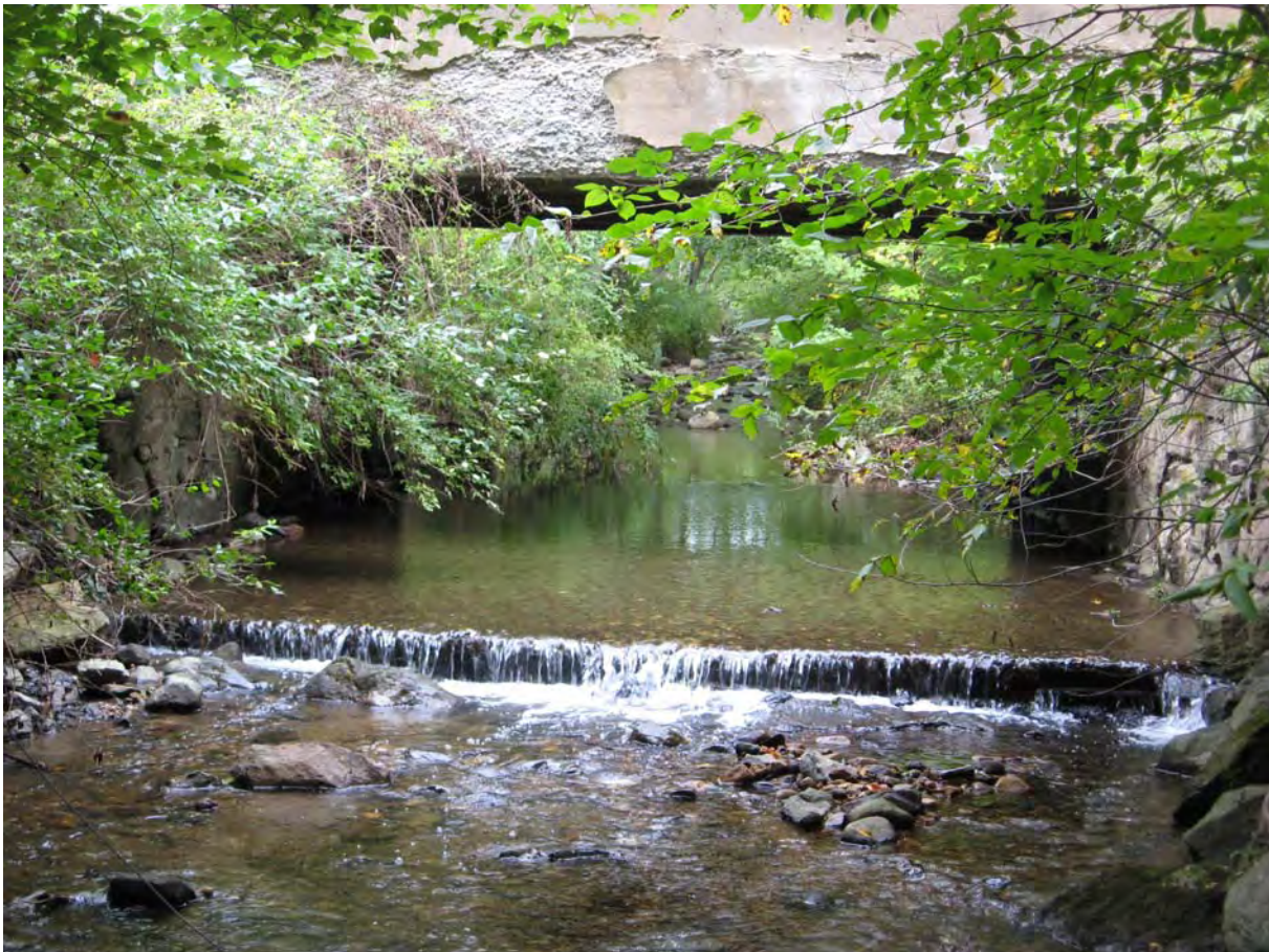
Figure 15: West Road Bridge Velocity Barrier
