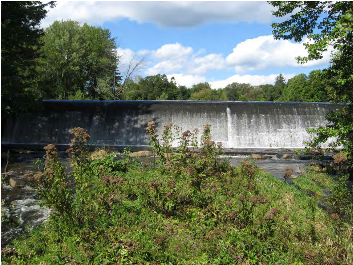
Figure 12: Heminway Pond Dam
