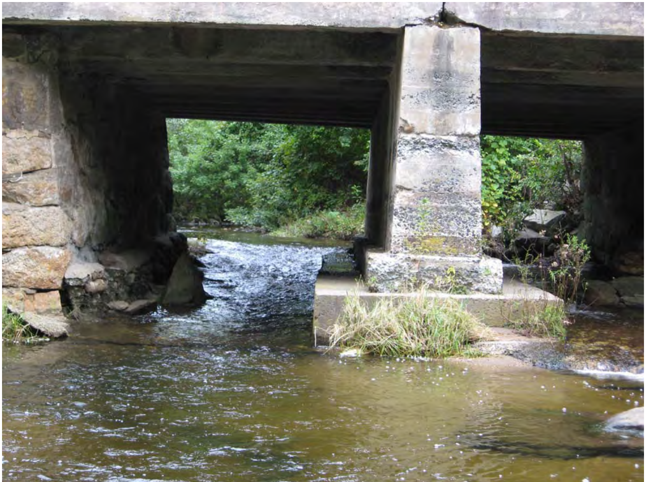
Figure 13: Northfield Road Bridge Velocity Barrier
