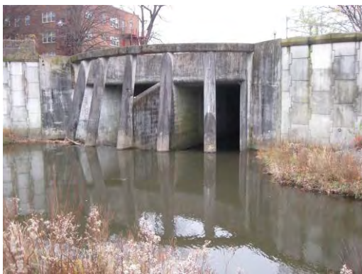
The North Branch Park River conduit entrance near Farmington Avenue.
