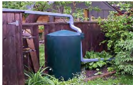
Rain barrel used to capture and re-use rooftop runoff (Source: CWP, 2007).
