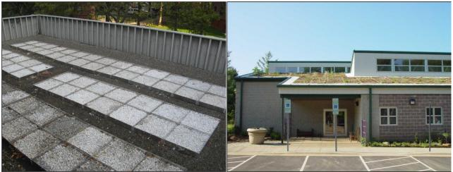
**Figure 4:** A blue roof consisting of engineered trays with stone ballast (left) and a green roof tray system installed on a sloped roof (right)
