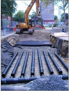
Figure 3: Subsurface chamber (top) and perforated pipe (bottom) infiltration systems under construction
