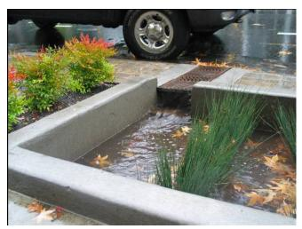
Figure 4.18 – Bioretention planters in Bridgeport, CT.
