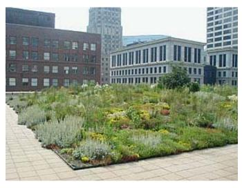
Figure 5.23 – Chicago City Hall green roof. Source: Photo (c) 2004 Roofscapes, Inc. Used by permission; all rights reserved.
