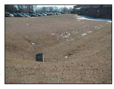
Figure 5.30 – Infiltration trench near a parking lot.
