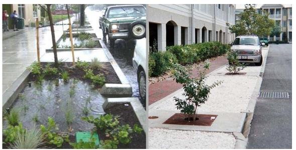
Figure 4.10 – Examples of planter box designs in high density development.
