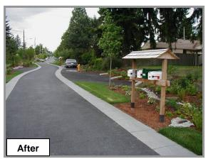
Figure 4.16 – LID urban retrofit project in Seattle, WA, using rain gardens/detention cells.
