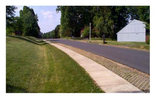
Figure 4.5 - Narrow road section with sidewalks, shallow swale and porous pavement shoulders.
