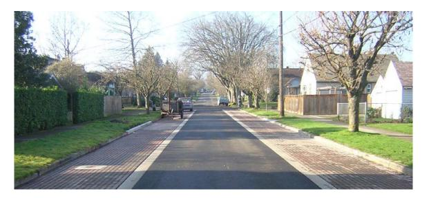
Figure 4.12 – Porous surfaces.
