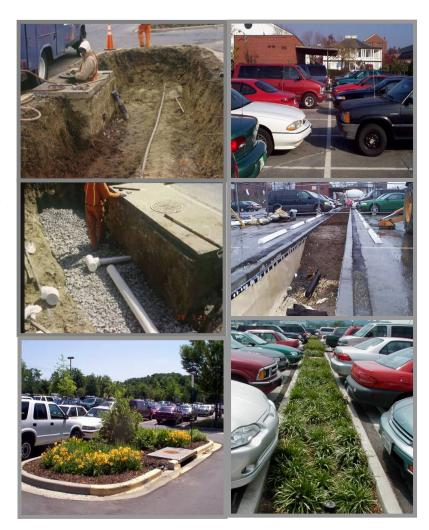
Figure 4.13 – Bioretention retrofit.
