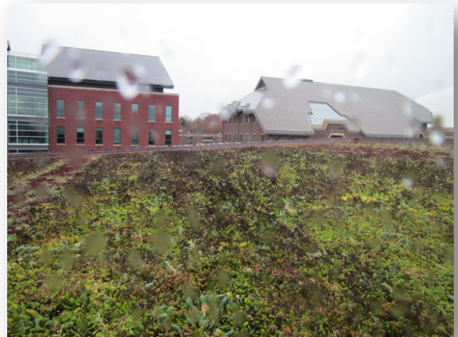
Green roof installed in 2011 at UCONN's new West Classroom Building. (Source: UConn CLEAR)
