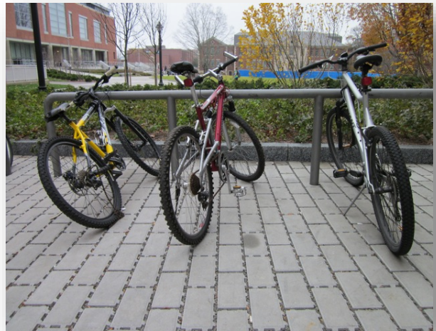
Porous pavers installed in 2011 at UCONN's new West Classroom Building. (Source: UConn CLEAR)
