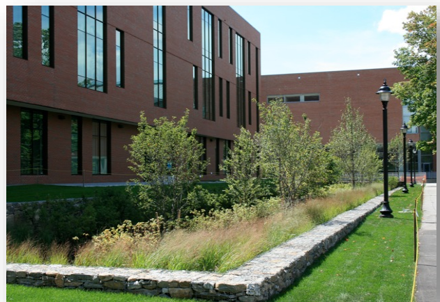
Bioretention swale installed in 2011 at UCONN's new West Classroom Building. (Source: UConn CLEAR)
