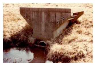
Concrete Intake Structure
