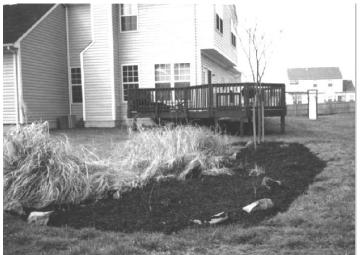
Figure 7.1. Even in the winter months, bioretention is effective for treating stormwater while providing visual interest.
