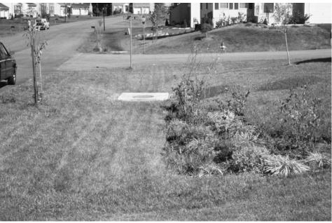
Figure 2.5. Swale-side bioretention
