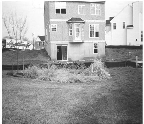
Figure 6.1. Silt fence around bioretention
