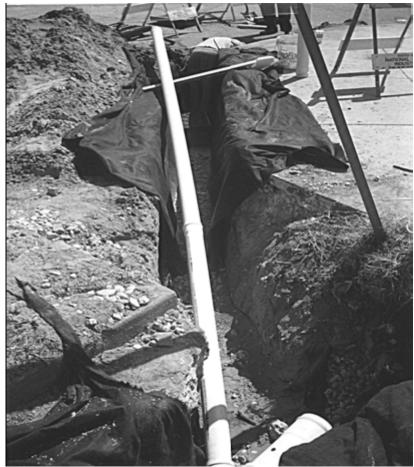
Figure 6.2. Installing an underdrain
