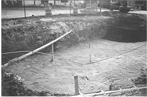
Figure 6.5. Natural compaction and settlement is recommended
