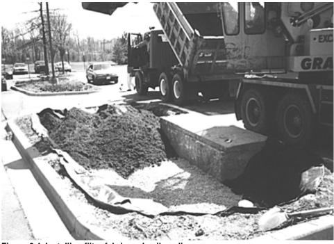
Figure 6.4. Installing filter fabric and soil medium
