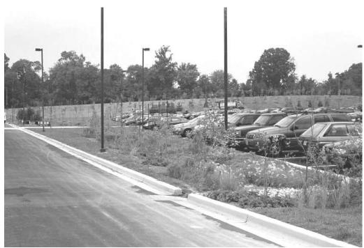
Figure 2.3. Curbed parking lot island and median bioretention
