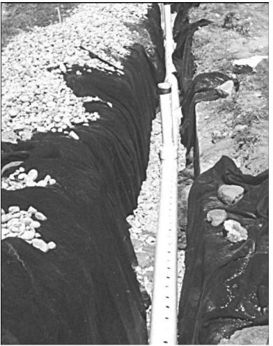
Figure 6.3. Installed underdrain pipe
