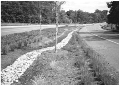
Figure 2.4. Median bioretention
