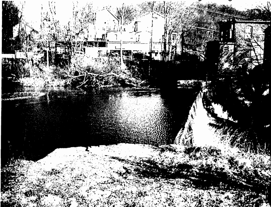
Photo 2-view looking northeast at concrete and stone dam for Pin Ship Pond. Buildings along Main Street are visible behind the pond.
