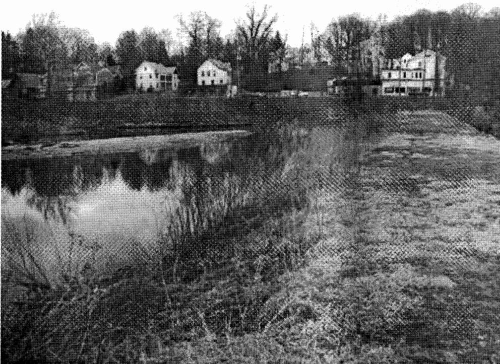
Dam – Pin Shop Pond (3/15/11).
