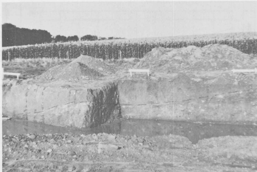
Fig. 8. A silty till, derived in part from varved clay, and overlying a compact sandy till; junction of Cedar and Willard Streets, Newington.
