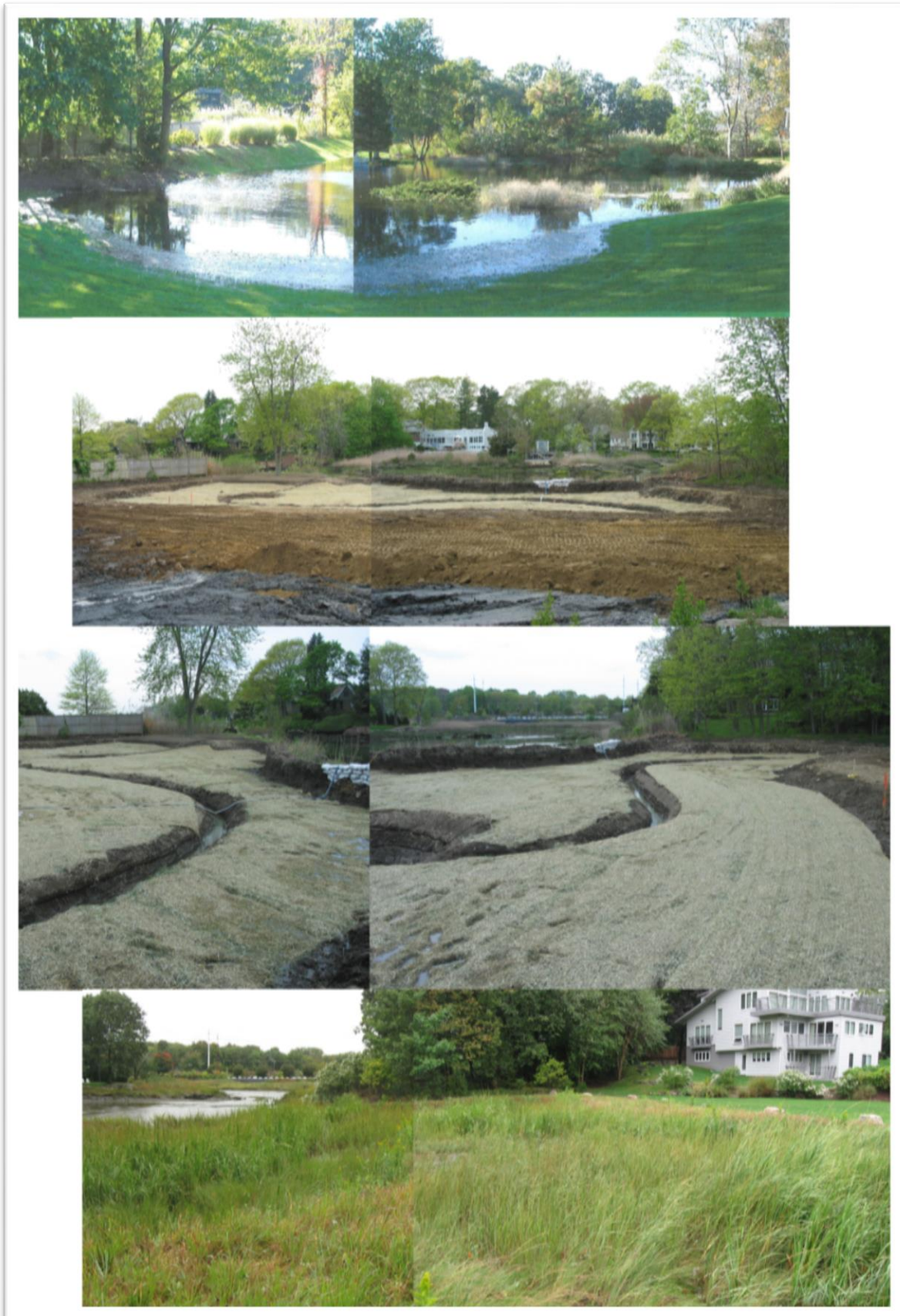
Figure 3. Restoration stages (top to bottom) at Burritt Cove, Westport
