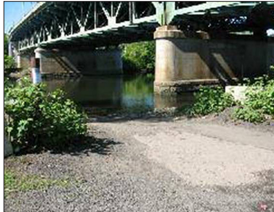
O'Sullivan's Island, Derby, CT. Site of bioremedial superswale.
