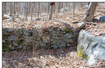
Corner of colonial dry-stone gristmill dam on Fort Hill Brook.
