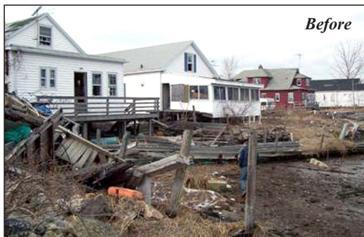
Long Beach West, Stratford, restoration.
