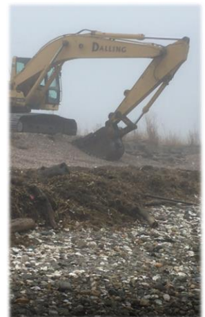
Dune construction at Stratford Point
