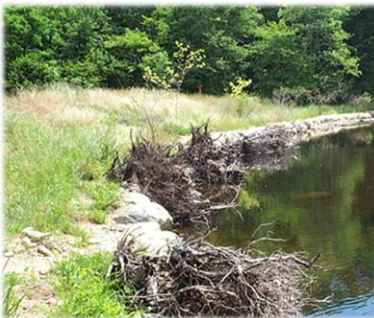
Root wads placed for bank stabilization on the Blackledge River, Colchester
