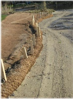
Coir logs staked for erosion protection
