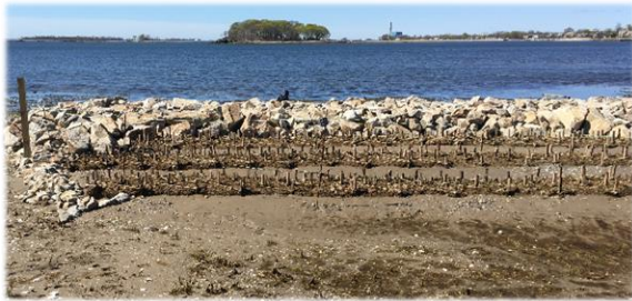
Riprap Sill protecting new tidal wetlands plantings in Westport
