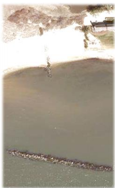
Offshore riprap breakwater at Fenwick Ave, Old Saybrook
