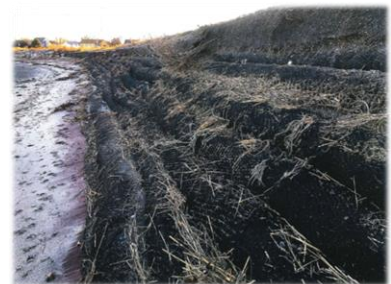
Geotubes used for dune creation at Stratford Point
