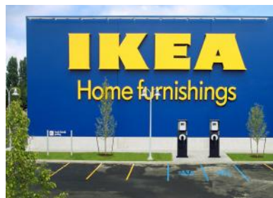
IMAGE 3. BURBANK, CA THE EVSE IS PLACED ON A CONCRETE PAD IN EXISTING LANDSCAPING, TAKING ADVANTAGE OF EXISTING OPEN SPACE IN FRONT OF THE PARKING SPOT WITHOUT REDUCING SIZE.
