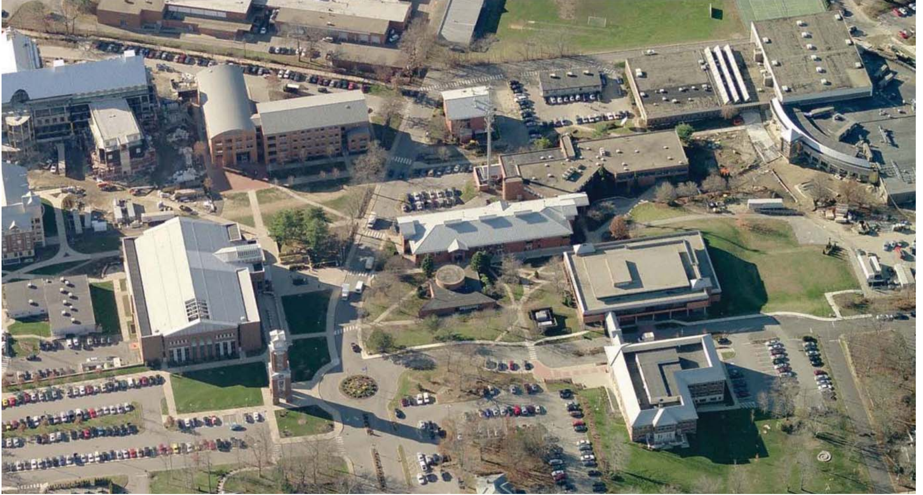
View of Central Quadrangle: Existing
