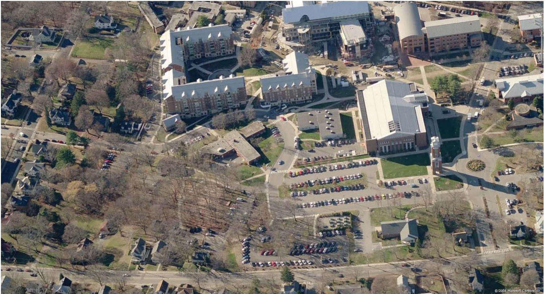
View of Clock Tower Road Quadrangle: Existing
