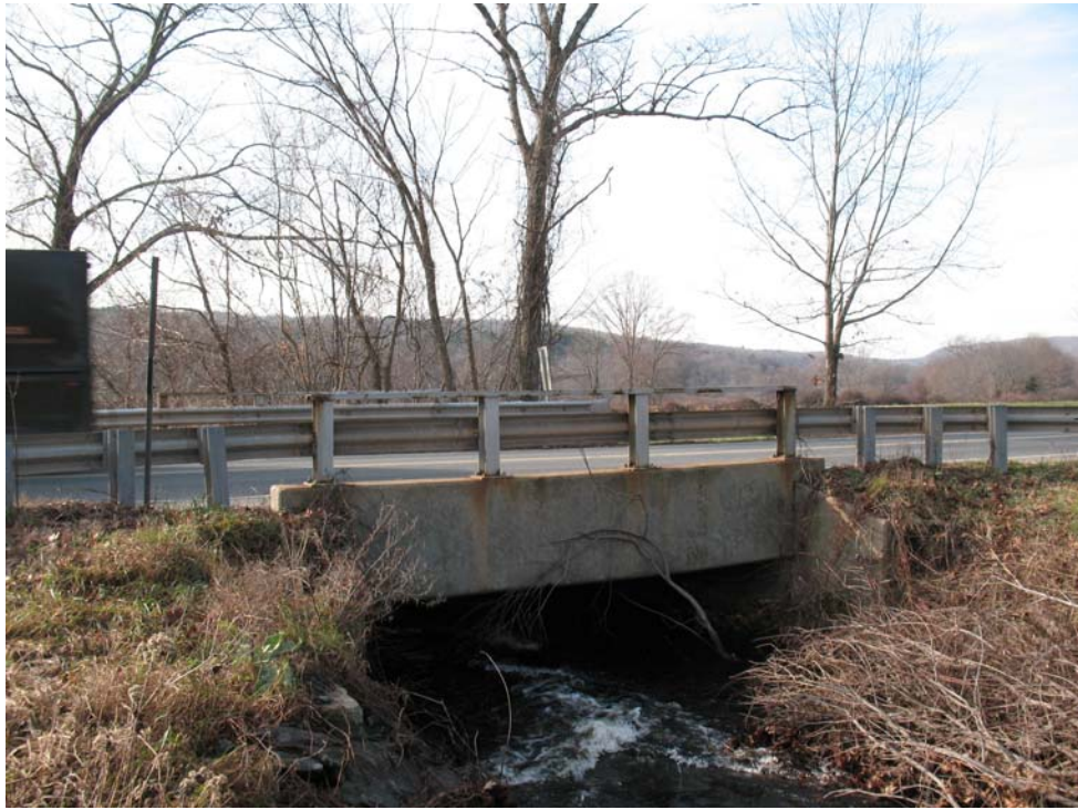
Pipeline Segment 55: Cedar Swamp Brook Culvert beneath Route 32
