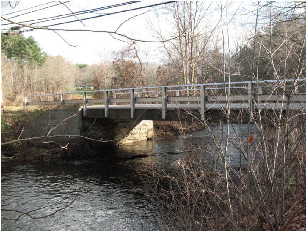
Pipeline Segment 36: Gurleyville Road Bridge over Fenton River
