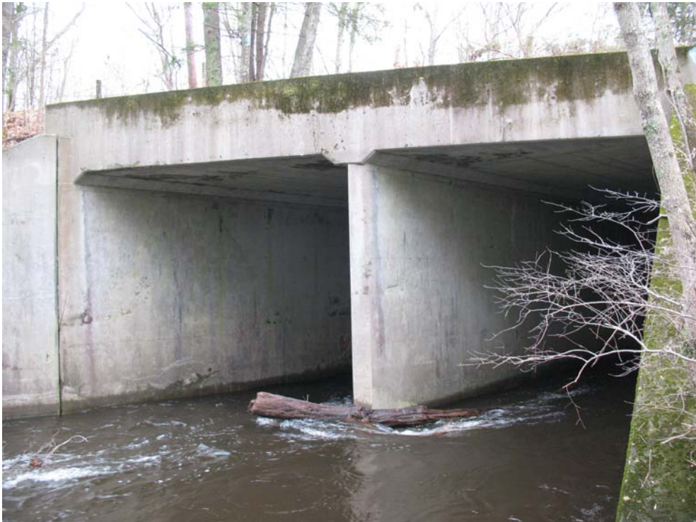
Pipeline Segment 35: Fenton River Box Culvert at Chaffeeville Road
