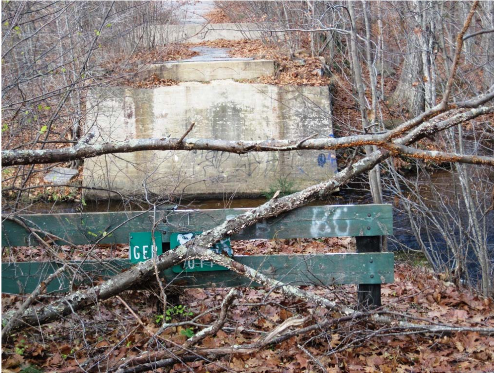
Pipeline Segment 12B: Former Bridge Abutment in Coventry Viewed from Mansfield
