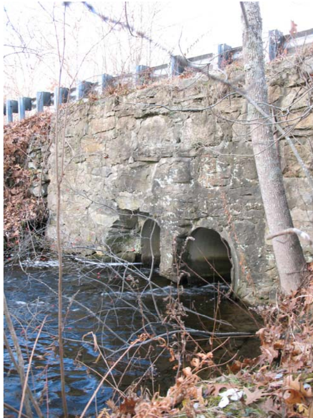
Pipeline Segment 39: Downstream Schoolhouse Brook Culvert on Clover Mill Road
