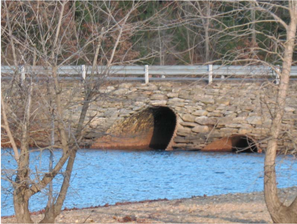
Pipeline Segment 23: Mansfield Hollow Lake Culverts beneath Bassetts Bridge Road
