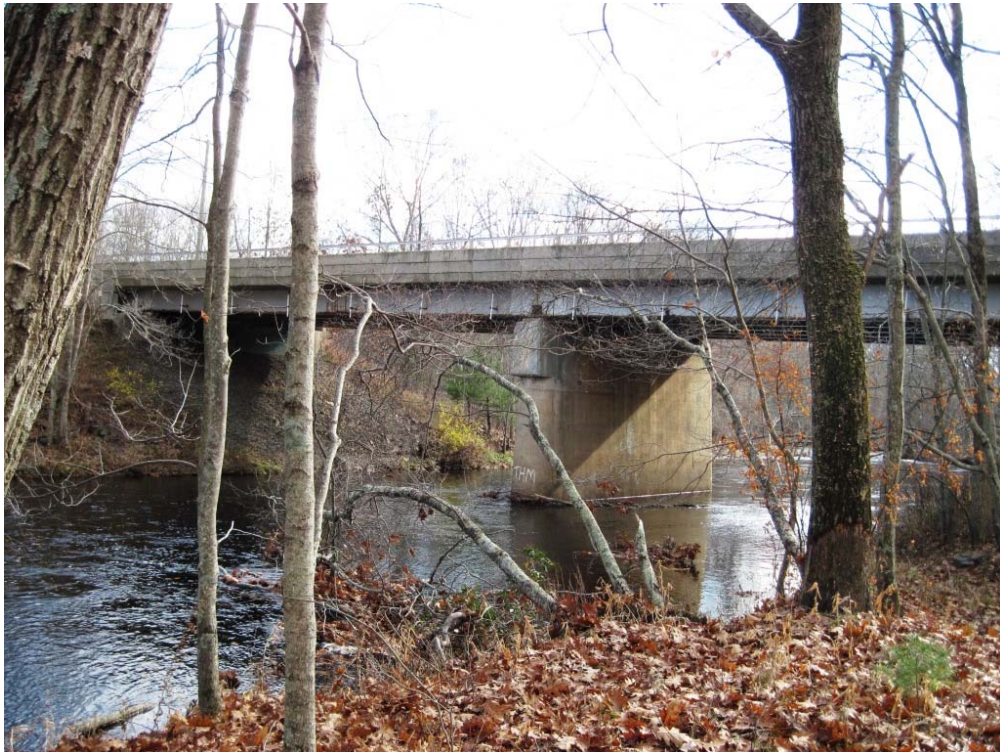
Pipeline Segment 12A: Route 195 Bridge over Willimantic River (Coventry/Mansfield)
