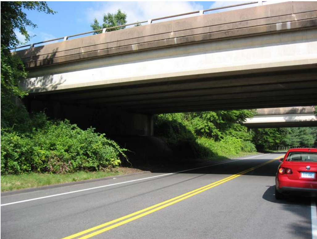
Pipeline Segment 2: Interstate 384 over Finley Street (Manchester)
