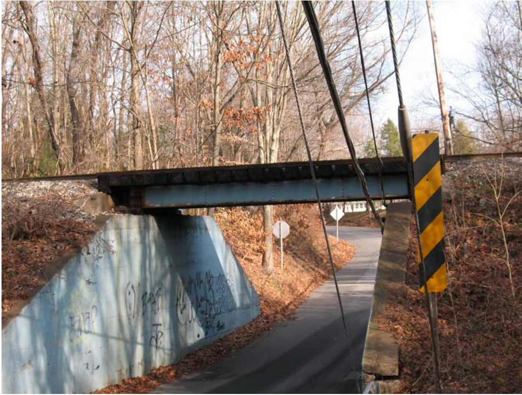
Pipeline Segment 42: Railroad underpass on Route 275 near Willimantic River
