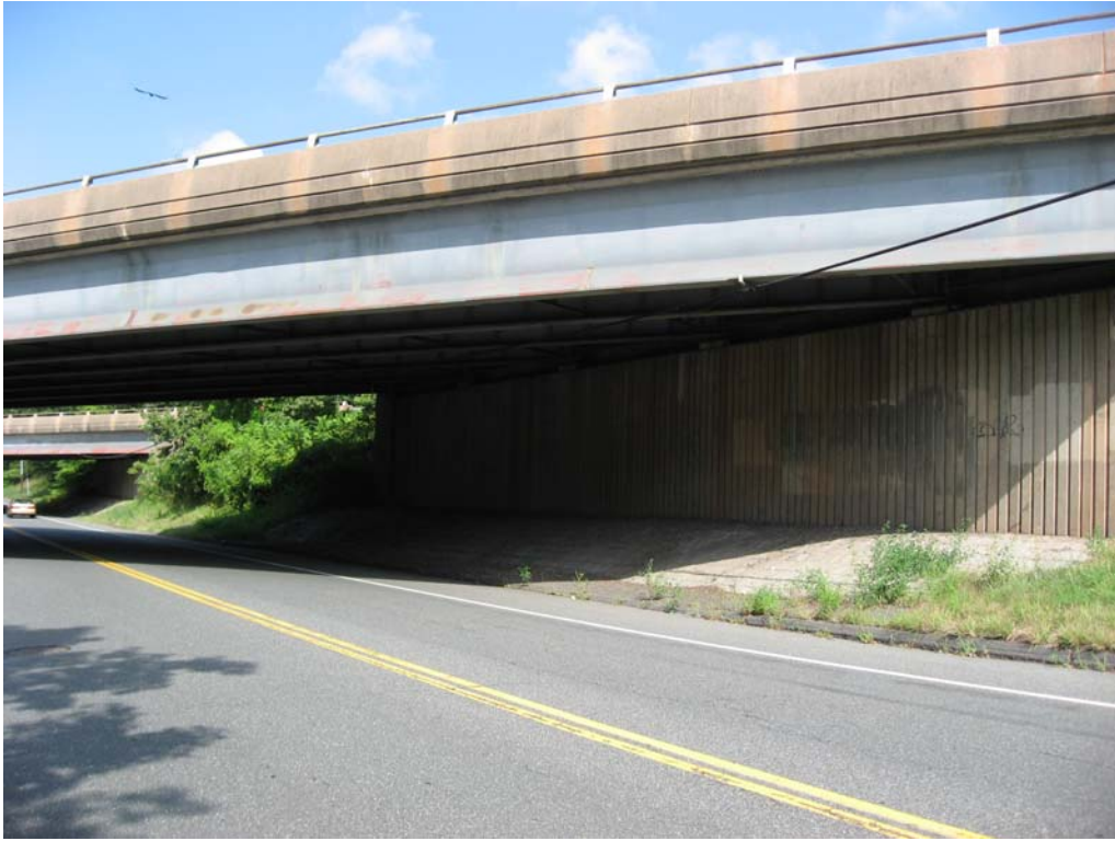
Pipeline Segment 2: Interstate 384 over Campmeeting Road (Manchester)
