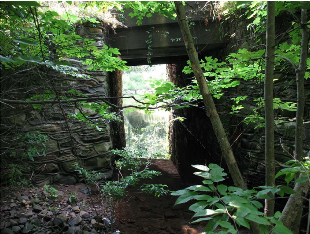
Pipeline Segment 2: Route 44 over Ash Brook (Coventry)
