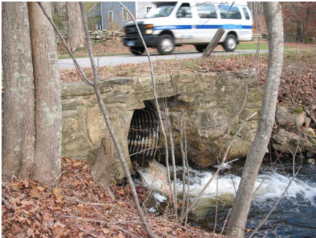
Pipeline Segment 39: Upstream Schoolhouse Brook Culvert on Clover Mill Road
