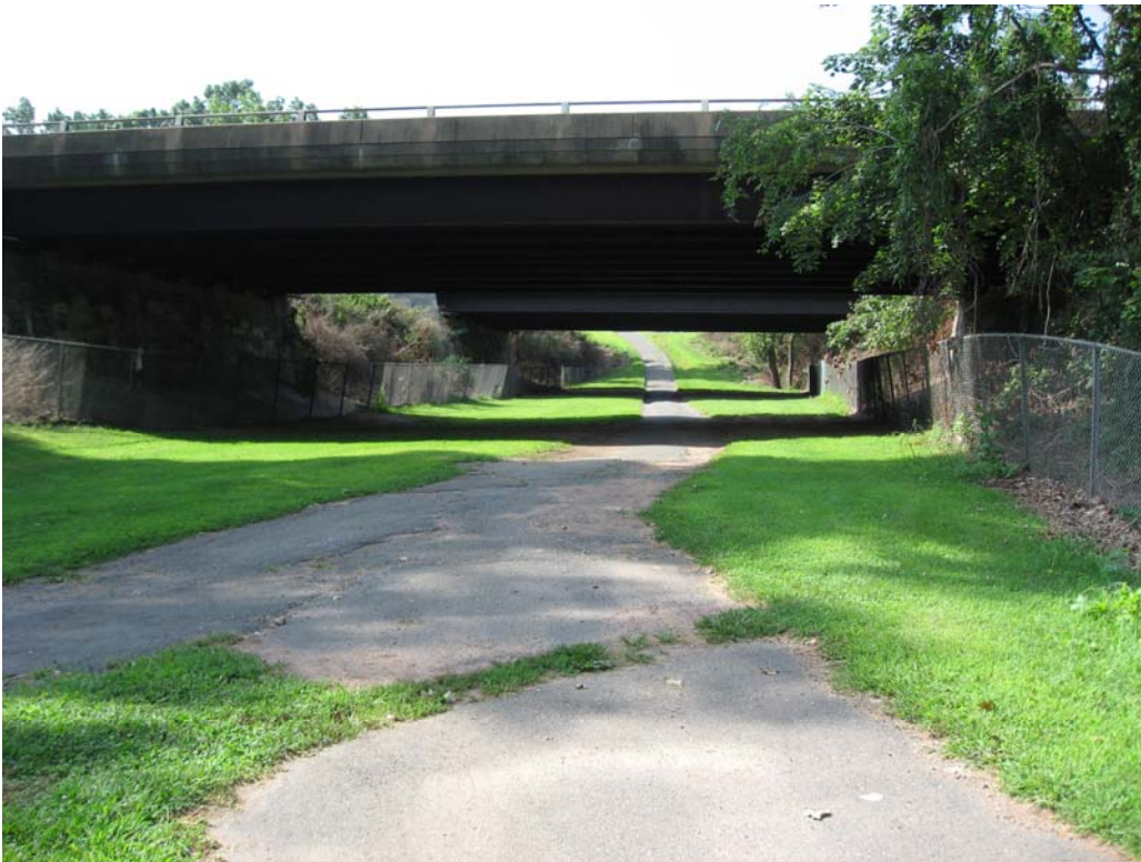
Pipeline Segment 2: Interstate 384 over Charter Oak Park Path (Manchester)
