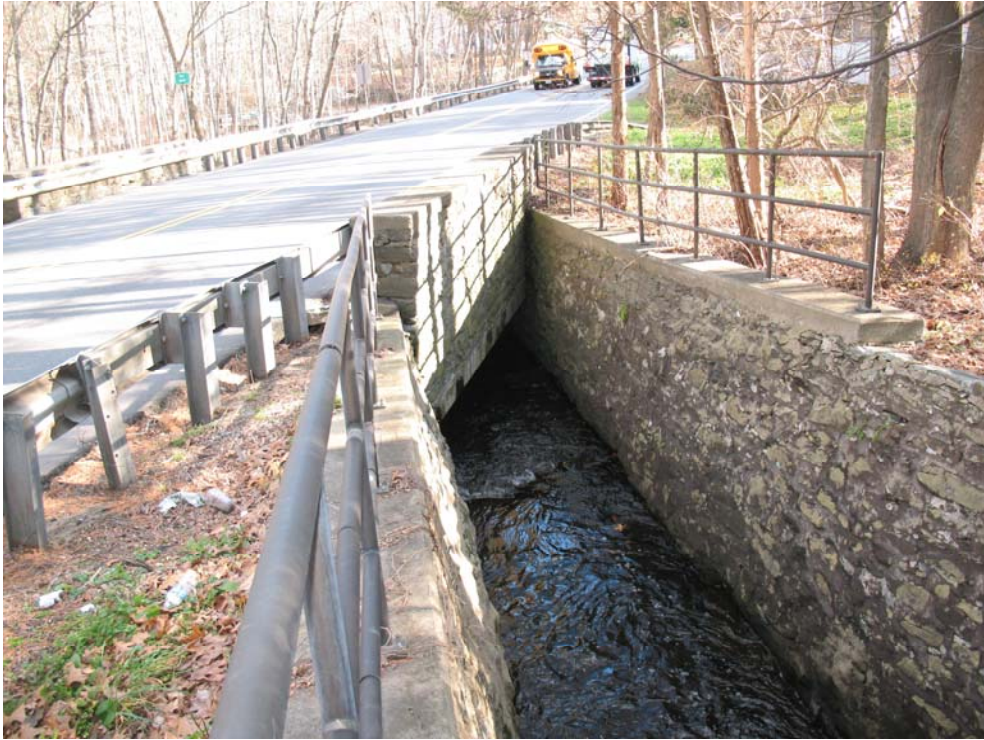
Pipeline Segment 34: Chapin Brook ("Mill Brook") Flume and Culvert beneath Route 195
