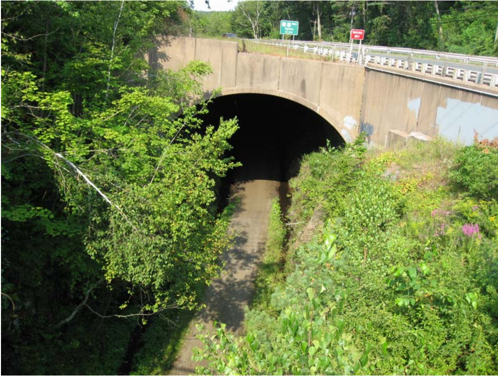
Pipeline Segment 2: Route 44 over Bolton Notch Linear Trail (Bolton)
