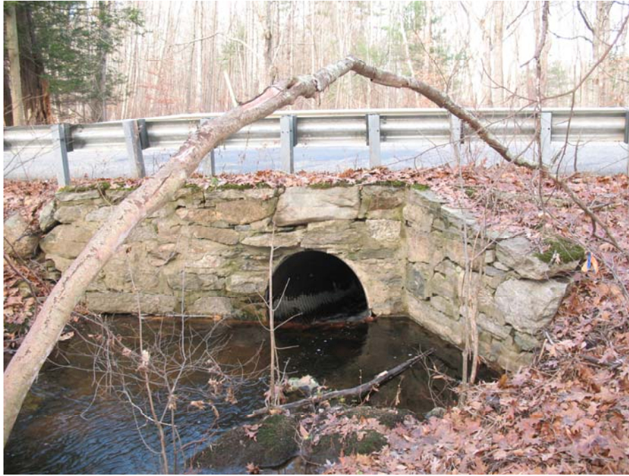
Pipeline Segment 39: Middle Schoolhouse Brook Culvert on Clover Mill Road
