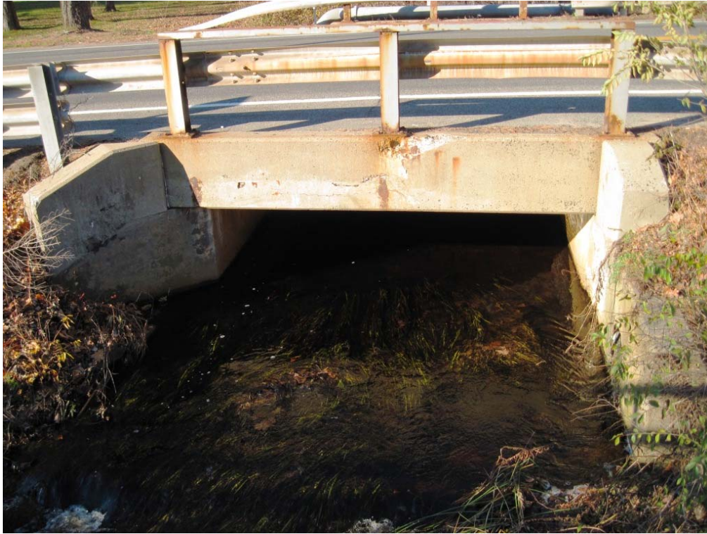
Pipeline Segment 18: Cedar Swamp Brook Culvert beneath Route 44
