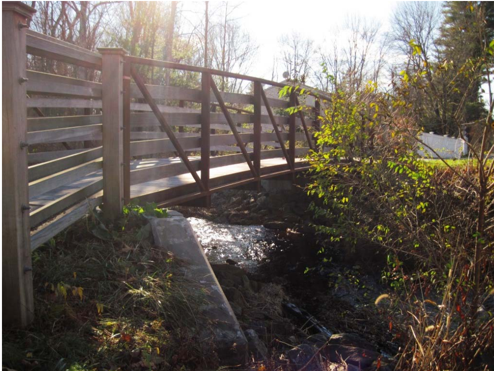
Pipeline Segment 18: Cedar Swamp Brook Pedestrian Bridge
