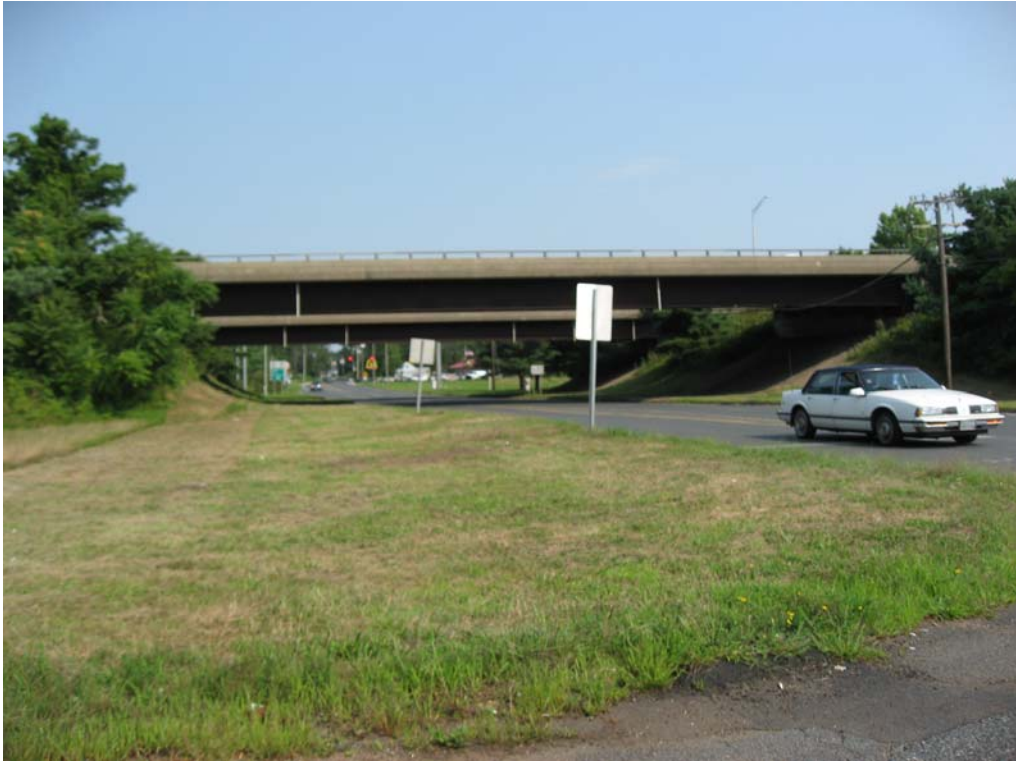
Pipeline Segment 7: Interstate 84 over Slater Street (Manchester)
