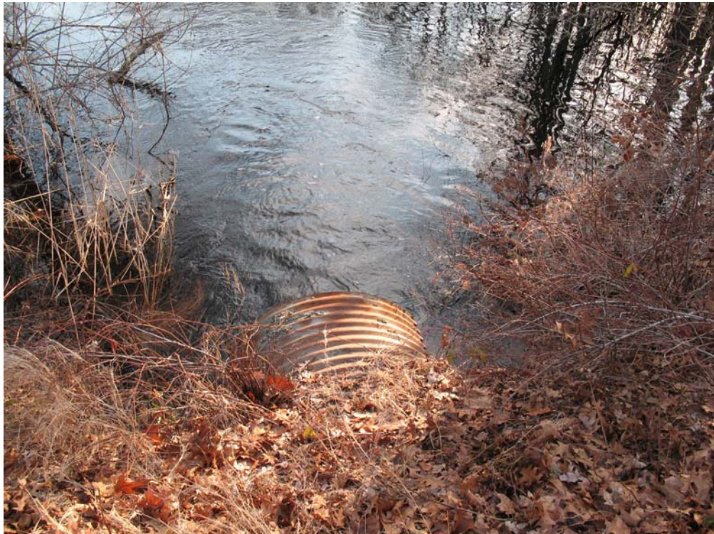
Pipeline Segment 14: Outflow Pipe from Cedar Swamp at Route 195
