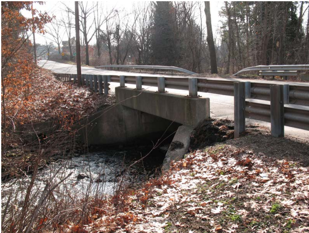
Pipeline Segment 52: Eagleville Brook Culvert beneath Route 32
