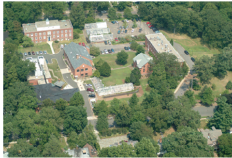
Main Laboratories, New Haven
