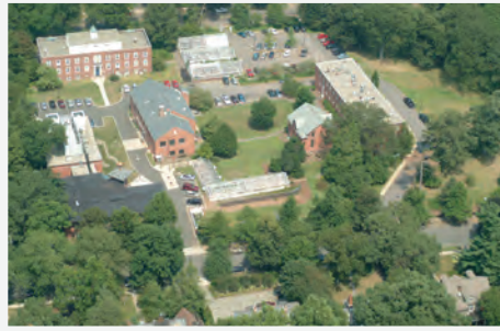
Main Laboratories, New Haven
