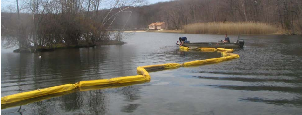
Figure 4. Installation of limnobarrier in Crystal Lake.
