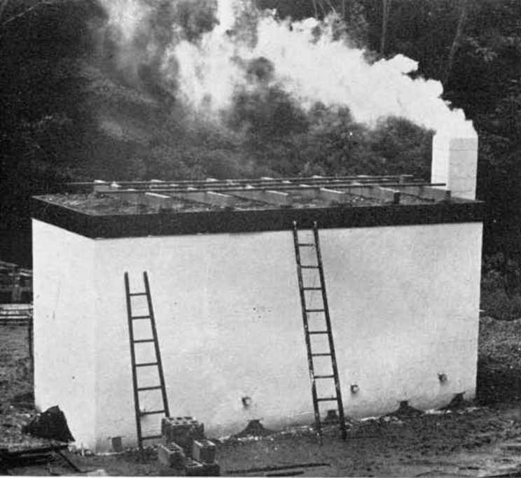
A seven-cord kiln in operation at Portland, Connecticut. In this case the roof is suspended from iron pipes laid on, and perpendicular to, six heavy timbers which span the walls. This kiln is end-fired and employs six air inlets on each side. The chimney is of cinder blocks for better insulation.
