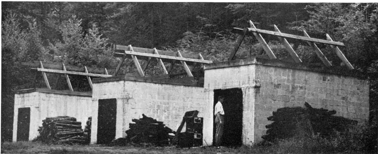
Three nine-cord kilns at Haddam, Connecticut. Note the open trusses which are a part of the suspensory system for the flat roof. The trusses may be covered with light sheet metal to protect the structure from rain or snow. These three kilns (estimated cost under $2,500), when operated as a battery, are capable of producing more charcoal per month than a 50-cord beehive kiln (estimated cost in excess of $6,000) which formerly stood on the same site.
