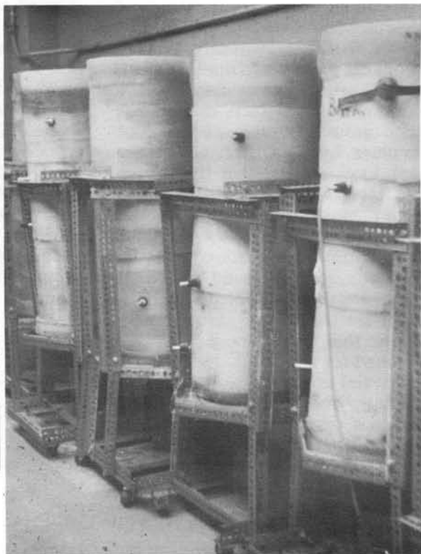
Undisturbed columns of soil, left, were encased in plastic, hoisted out, and taken to the Soils laboratory in New Haven.
