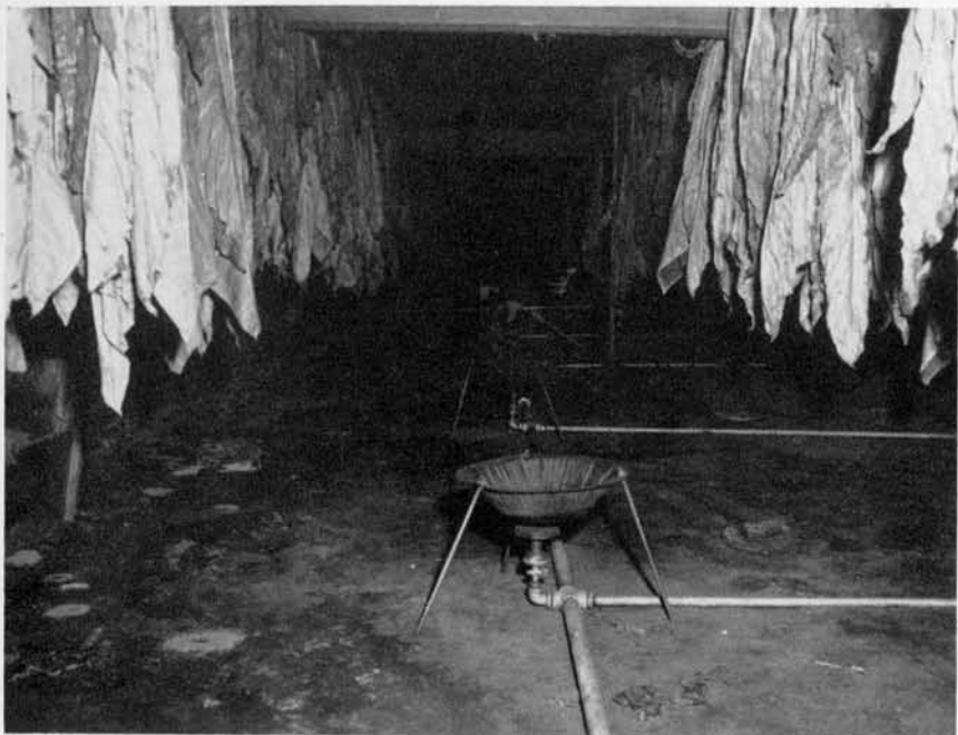
Figure 10. Improvised gas stove using a manufactured burner part and a charcoal pan for heat deflection. This type was moderately successful in the shed of Broadleaf shown here. Note absence of rubber hoses. See Figure 5.
