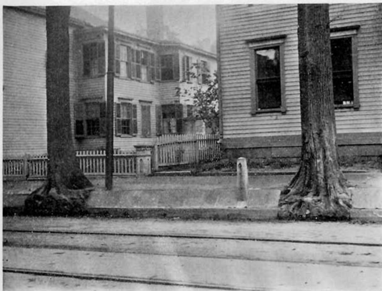
Fig. 3. —Trees mutilated in laying curb and gutter.
